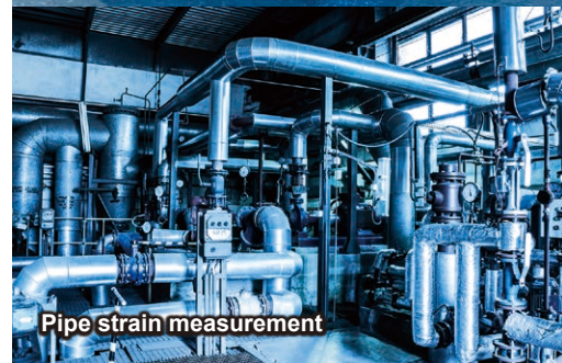
Brake and pipe strain measurement
